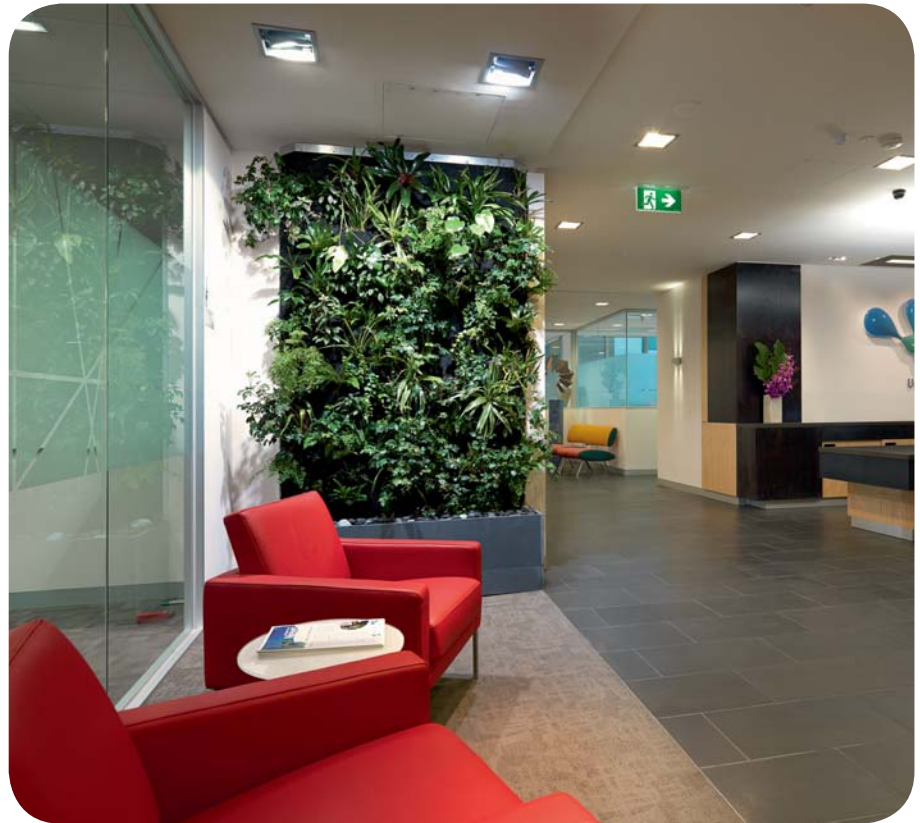
Five bio-filtration walls remove volatile organic compounds from the air.
