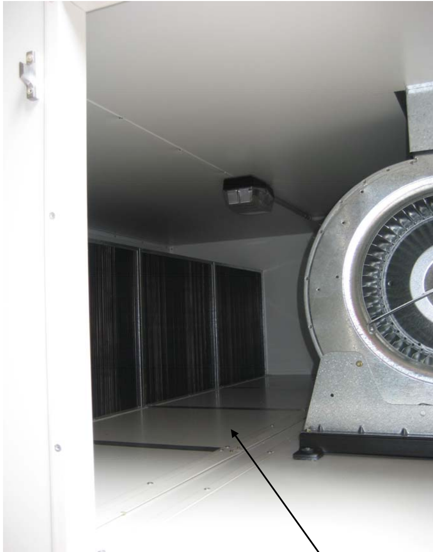
Removable Panels for Coil Access
