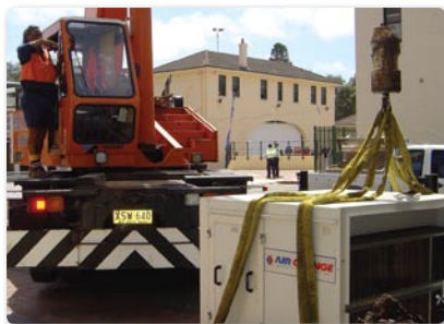
Lifting the Air Change Package Unit into the roof of the Bondi Pavilion
