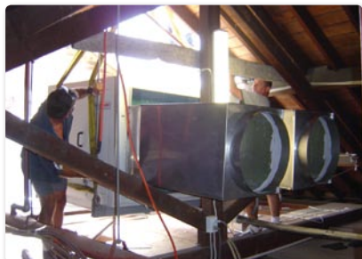
The Air Change ACS 16 being lifted into position by Rob & Chris showing the exhaust air trouser piece either side of the roof timber post
